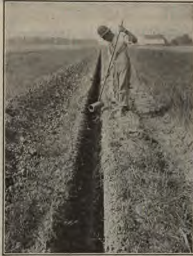
FIG. 201. — Laying tile in ditch.
